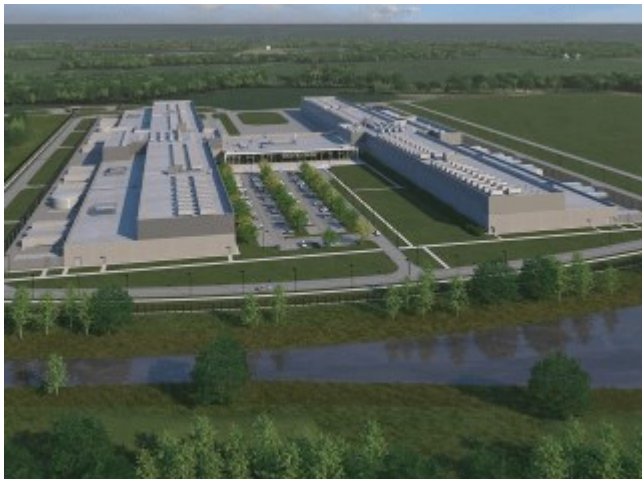
Facebook's New Albany, Ohio, Data Center This is the image that New England Edge recommended the Town Council look at to get an idea of what data centers look like.
